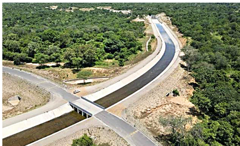
Figure 10: Main Canal – Shire Valley Transformation Project in Southern Malawi
